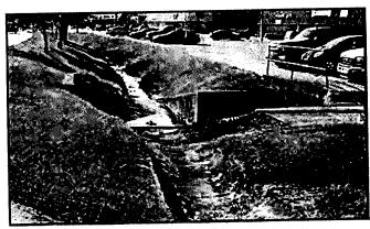
and improve water quality. By enclosing the area were numerous pipes converge a pedestrian hazard would be eliminated and the area aesthetics can be improved. This area would be designed with an overflow structure to assure flooding does not occur during large storm events.
