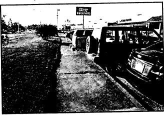
The drainage issues on Southland Drive are similar to those throughout Lexington. With ditches that have extremely flat grades and inadequate detention for the impervious pavement, flooding is a result. Although this project cannot solve all the drainage issues, it does offer the opportunity to improve existing conditions by providing properly sized pipes and improving the ditching.
