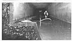
After issuing an "Urgent and Compelling" status due to the instability of these 1940s outfall structures, USACE hired URETEK to stabilize both the Addicks and Barker Reservoirs. URETEK's unique process stabilized both outlet structures in less than three weeks making them structurally stable, safe and capable of staying in sevice for the City of Houston and surrounding communities.
