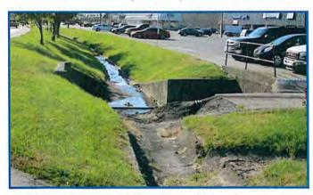
and improve water quality. By enclosing the area were numerous pipes converge a pedestrian hazard would be eliminated and the area aesthetics can be improved. This area would be designed with an overflow structure to assure flooding does not occur during large storm events.
