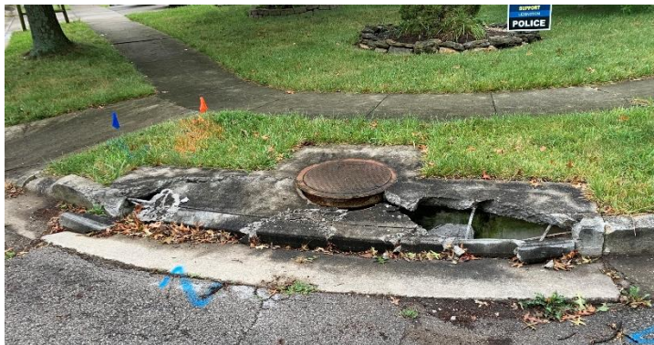
Completely Broken Inlets
