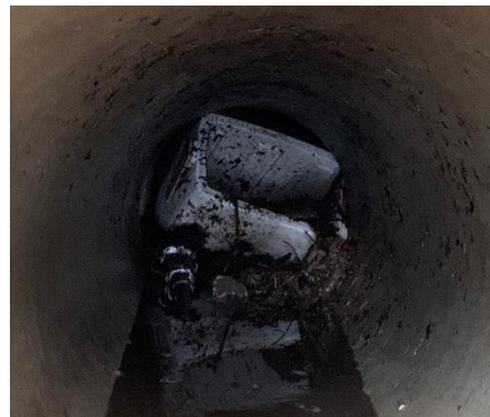
Coolers blocking Storm Pipes
