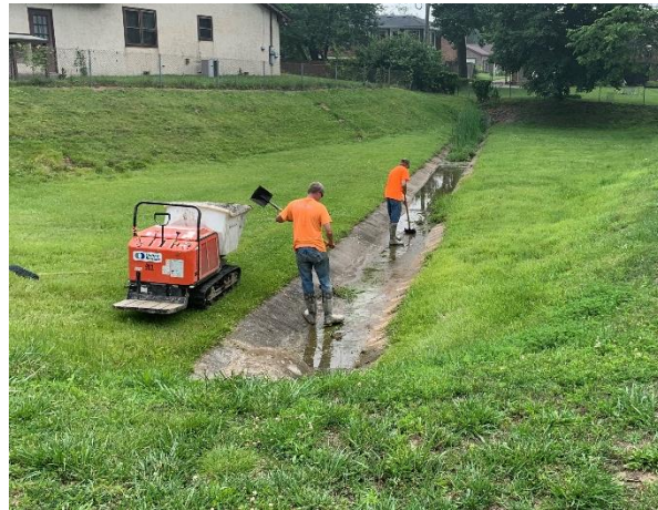
Cleaning Concrete Flumes
