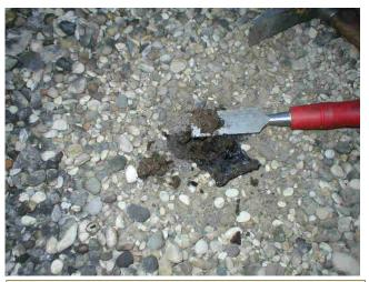
B) Area #2 Core Cut -Saturated Perlite Insulation
