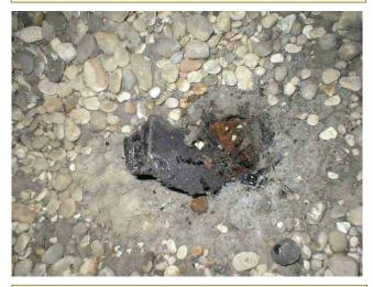
C) Area #5 Core Cut -Saturated Fiberboard Insulation
