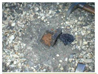
A) Area #1 Core Cut -Saturated Fiberboard Insulation
