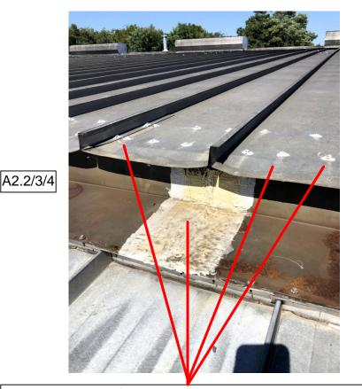
Note: Example of existing sealants to be removed. Replace 3 course details in similar manner. Replace sealant at all fasteners.
