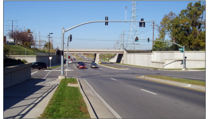
West Reynolds Road Railroad Underpass Reconstruction.
