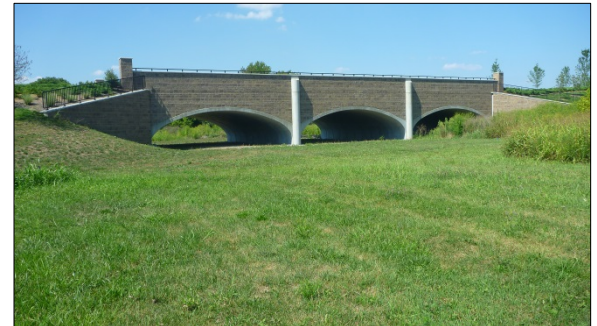
Eastern State Hospital ConSpan Arch Bridge.
