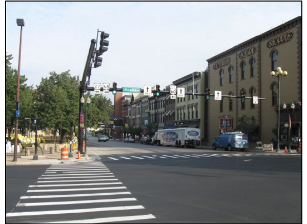
West Main and Broadway Traffic Signal During Construction.
