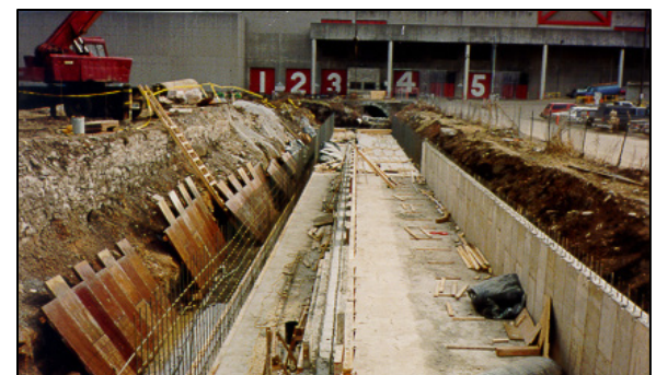
Heritage Hall Expansion - Chambered 12-foot x 6-foot storm and 5-foot x 4-foot sanitary R.C. Box Culvert - Upstream Town Branch Creek.
