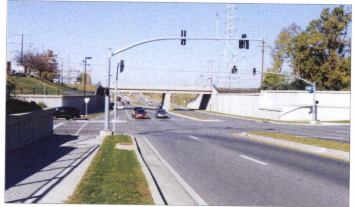
West Reynolds Road Railroad Underpass Reconstruction.
