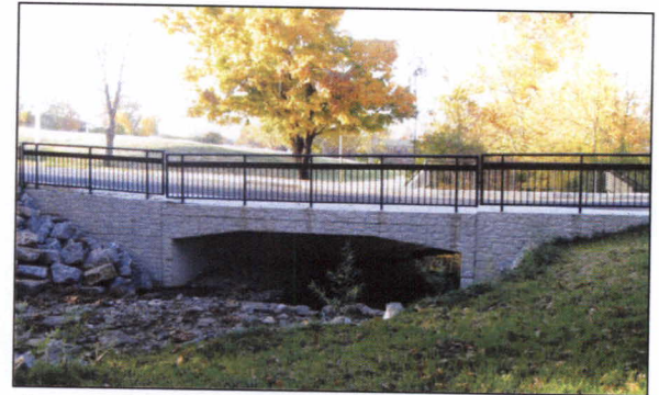
Appomattox Road Culvert Replacement 24-foot x 6-foot R.C. Box Culvert.
