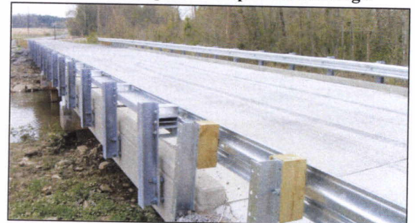
Bean Cemetery Road Bridge Replacement. Madisonville, KY.
