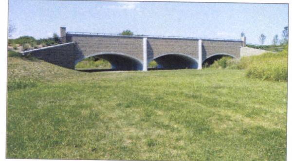
Eastern State Hospital ConSpan Arch Bridge.
