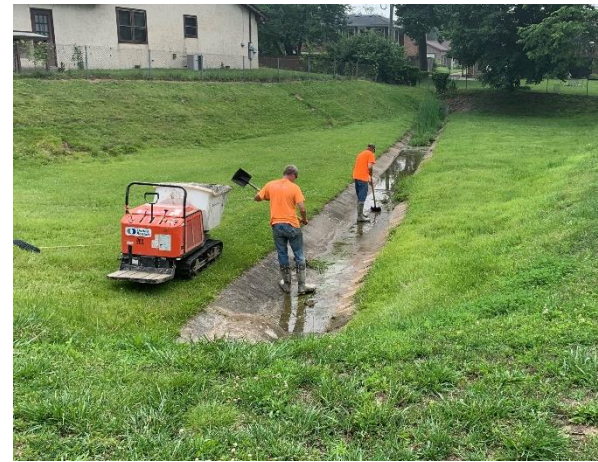
Cleaning Concrete Flumes
