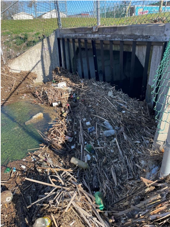
Edgelawn Detention Basin (After Big Storms – Help (as-needed))
