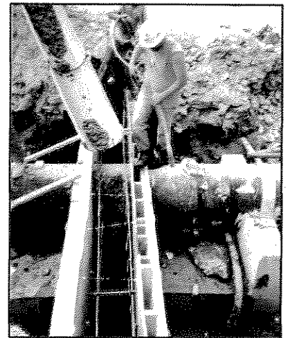
Expansion Area 2C 30-in Trunk Sewer Reservoir Crossing - Lexington, KY
