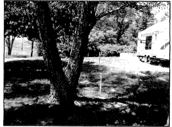
Ashgrove Mobile Home Park Sewer Line - Field Alignment Review.
