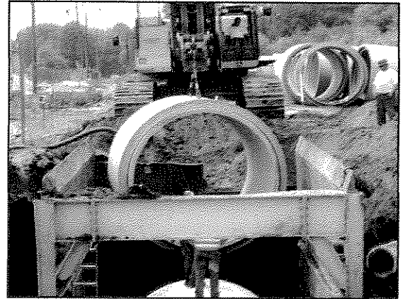
Noblitt Park 66-in. Sanitary Sewer Interceptor - Columbus, IN
