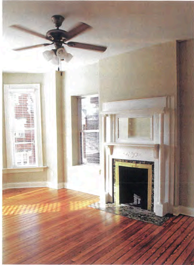
Photo Courtesy: AU Associates Inc. AU Associates Inc. restored the original mantels and floors at the First Presbyterian Church Apartments.
