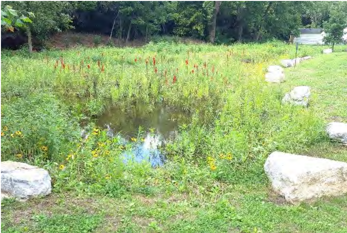
The WGPL WQ Basin includes native plantings, bioretention, and boulders marking the no-mow zone.
