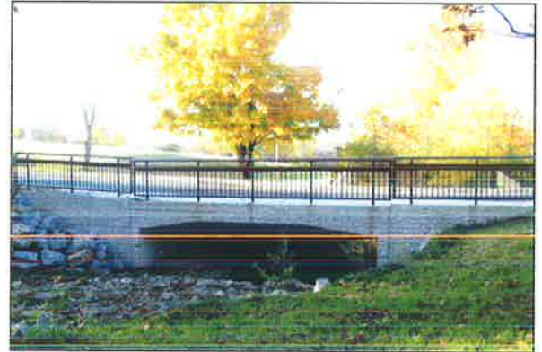
Appomattox Road Culvert Replacement - Double 12-foot x 6-foot R.C. Box Culvert.
