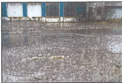
Storm sewer surcharge of street inlet and street flooding on Trafton Street after heavy rainfall
