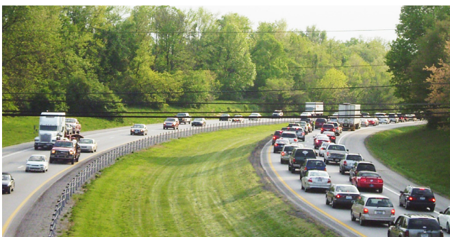
I-71/I-265 Interchange, Jefferson County, KY.
