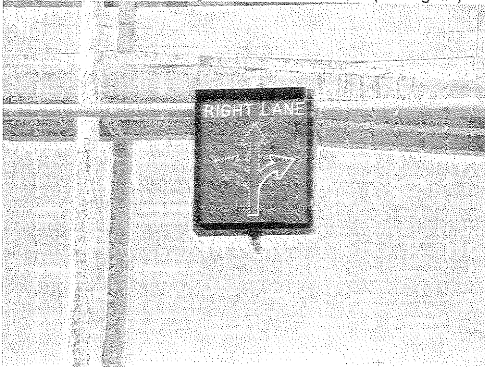
LED Lane Use Control Signal, 30-inch x 36-inch, #2 (Message #1)
