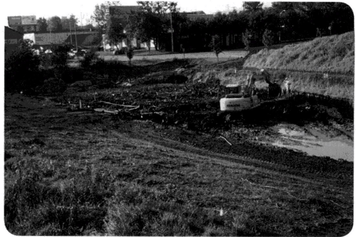
Installation of gravel/wood chip aquifer at MMSK Stream project in Lexington.
