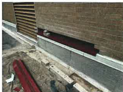
RPC – Masonry Repairs
