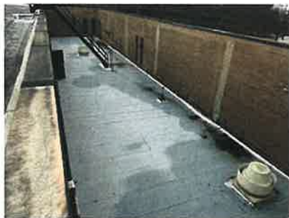
Tech 'A' - Roof
