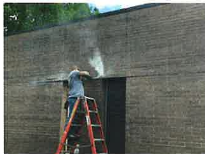
Tech 'A' - Masonry
