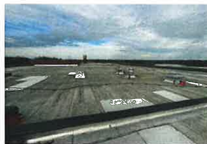
ATB – Roof Repairs
