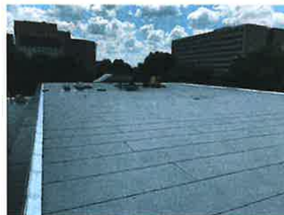
Tech 'B' - Roof
