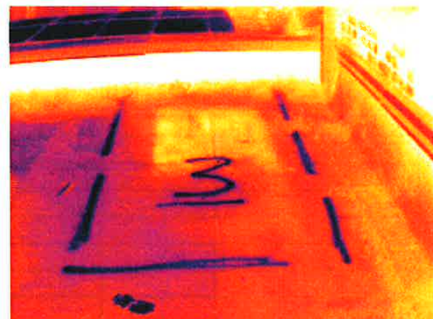
Infrared view of area #3
