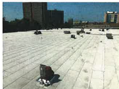
Tech 'B' - Roof
