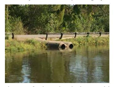
The section of roadway to be widened is surrounded by the Kentucky American Water Company reservoir and has pipes running beneath it. It is the desire of LFUCG to widen the roadway to accommodate the passage of two, large emergency response vehicles. In order to accomplish this task, the loading capacity of the roadway is to be evaluated and methods for increasing capacity are to be made, if needed.
