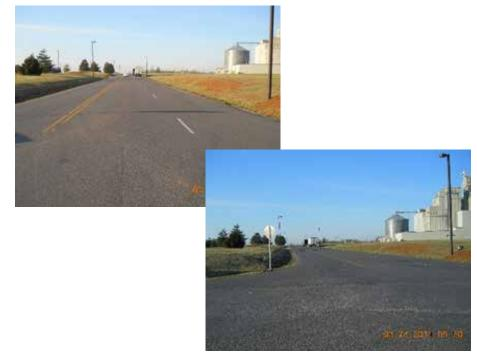
This project consisted of constructing an additional 6' width on each side of Quintin Court in the industrial park in order to widen approximately 1000 lf of roadway from 2 lanes to 3 lanes. The project also included drainage. Continuous truck traffic was maintained through the site, as was required by the adjacent mill. Coordination with existing utilities was required for lighting and relocation of a water main.
