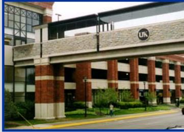
The structures utilized two precast prestressed concrete type III I-beams in the cross-section. This design proved to be a challenge because the beams over Limestone cantilever past the support pier positioned away from the garage. The cantilever was an effective solution that allowed the foundations of the garage and bridge to remain independent. The design required unusual strand configurations to accommodate the stresses produced in the cantilevers.
