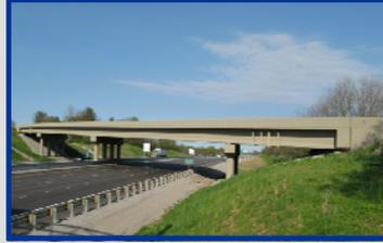
A high skew of 45 degrees and multiple spans with limited vertical clearance over I-64 also made this design a challenging project. Due to the skew, expansion abutments on steel H-piles were required. The three multi-column piers were founded on spread footings on rock.
