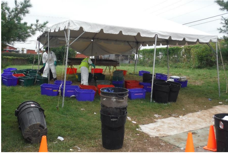
Figure 2-1 Work Area at Bluegrass Transfer Station
