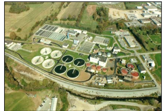
Town Branch WWTP.
