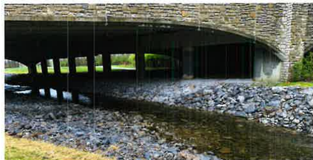
Cane Run Bank Stabilization (Before/After) – Lexington, KY
