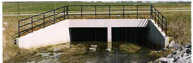
Wellington Development Box Culvert – Lexington, KY
