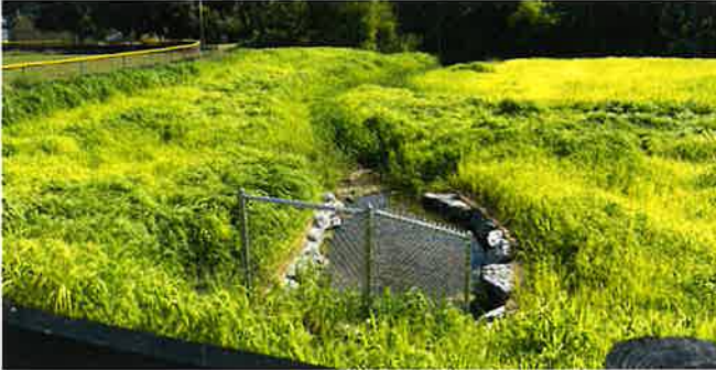
Southland Park Stormwater Control Basin – Lexington, KY
