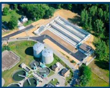
The Equalization Basin in Napoleon, Ohio was located in the 100-year floodplain for the Maumee River and designed to prevent floatation and resist hydraulic uplift forces.
