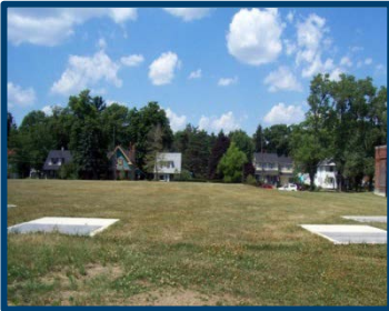
The River Road Equalization Basin included a concrete tank located below a public park in Toledo, Ohio. The project is part of the City remedial measures capital program to meet the requirements of their EPA Consent Decree.
