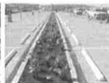
Parking Lot Bioretention
