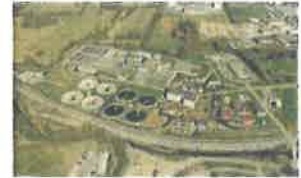
LFUCG's 30-mgd Town Branch WWTP
