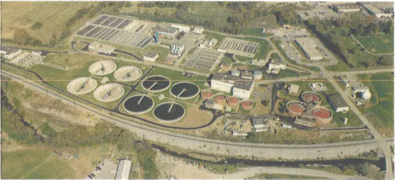
Town Branch Wastewater Treatment Plant.
