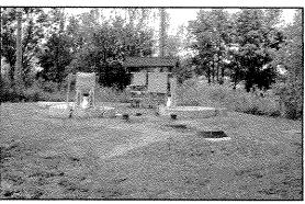
The Spindletop Pump Station, with split wetwell design, emergency pump connection and provision for emergency generator.
