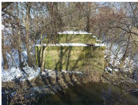
Existing stone abutments were reused for prefabricated steel truss bridge.
