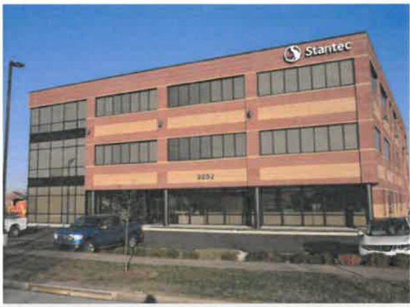
Stantec's Lexington office at 3052 Beaumont Centre Circle
