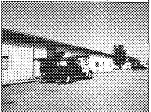
Photo of Approx. Sounding Location
