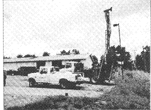
Photo of Approx. Sounding Location
