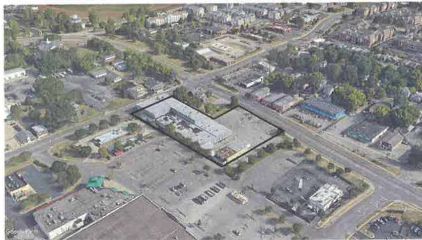
View Looking North
