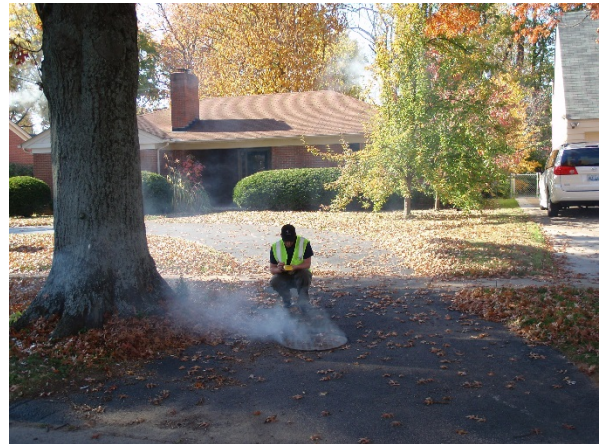
The information we collected during the Sanitary Sewer Assessments is aiding in identifying capacity-earning opportunities.
