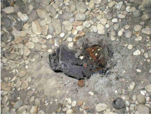
C) Area #5 Core Cut -Saturated Fiberboard Insulation
