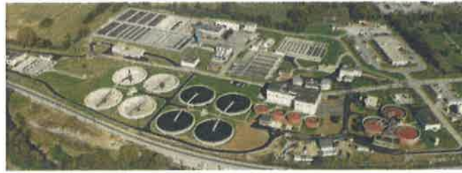
Town Branch Wastewater Treatment Plant.
