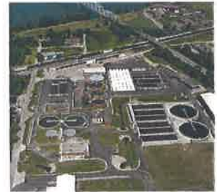
Parkersburg Utility Board's 19th St. WWTP.
