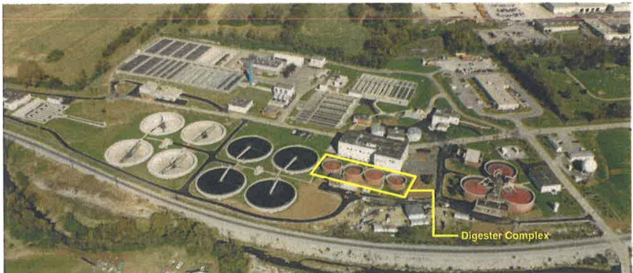
Town Branch Wastewater Treatment Plant.
