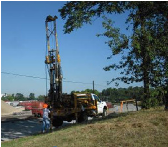
Newtown Pike extension drilling
