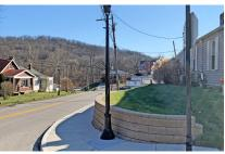
**Main Street Sidewalks, Kenton County, KY** - The City of Bromley engaged Palmer Engineering to design sidewalk improvements along Main Street and design of a pile and lag retaining wall. The existing retaining wall had failed, resulting in the sidewalk having to be closed. Right-of-Way services involved 2 acquisition parcels.
