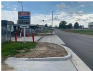
Due to the high cost of relocating utilities, special consideration was taken to minimize utility impacts. As a result of the detailed design, no utilities impacted the project. An example of mitigating utility impacts, the drainage design utilized overland flow and curb and gutter flumes, contrary to a more expensive underground storm sewer.
