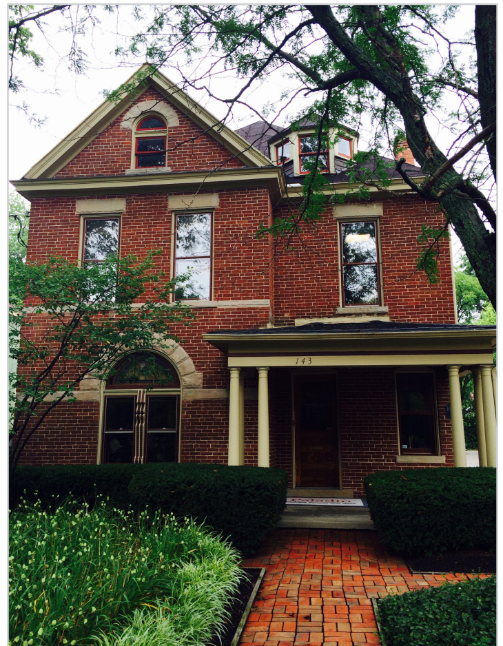
Paladin's Offices are located at 143 Walton Avenue in Lexington
