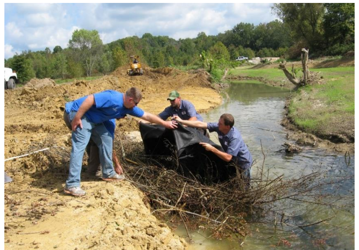
Casey Mattingly oversees installation of brush and woody debris
