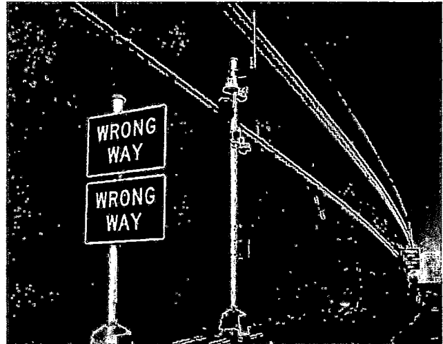
ITS equipment along a highway
