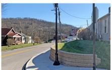
**Main Street Sidewalks, Kenton County, KY -** The City of Bromley engaged Palmer Engineering to design sidewalk improvements along Main Street and design of a pile and lag retaining wall. The existing retaining wall had failed, resulting in the sidewalk having to be closed. Right-of-Way services involved 2 acquisition parcels.
