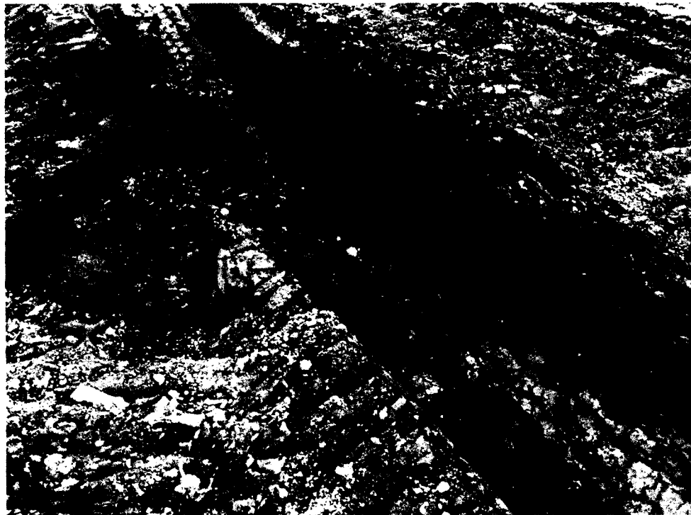
Photo 6: View Of Ruts After Proof Roll
