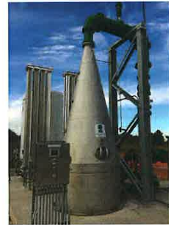
ECO2 superoxygenation system. Offers a high level of odor control in a compact footprint with relatively low yearly operations costs.
