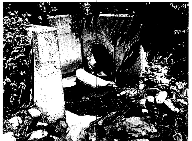
OUTFALL STRUCTURE—120HW (Note staining on rock channel)
