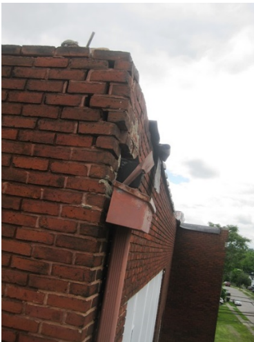
North corner of Roof Area 1
