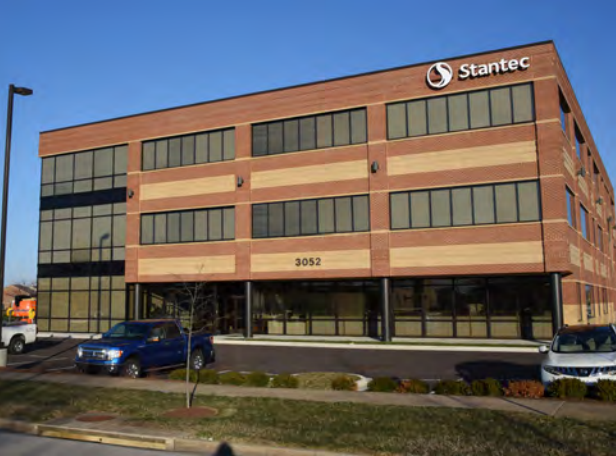
Stantec's Lexington office at 3052 Beaumont Centre Circle
