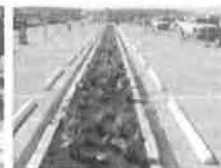
Parking Lot Bioretention
