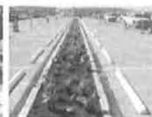
Parking Lot Bioretention
