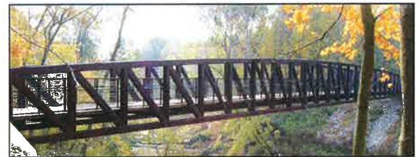
Ohio River Levee Trail.
