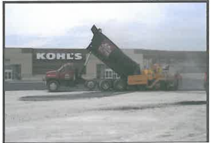
Excavation/Rock Installation&Paving@Kohl's
