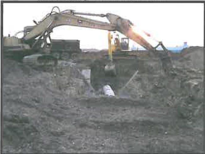
Storm Drainage work at Fayette Mall
