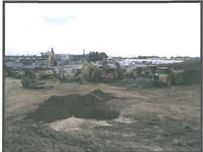
Excavation at Fayette Mall
