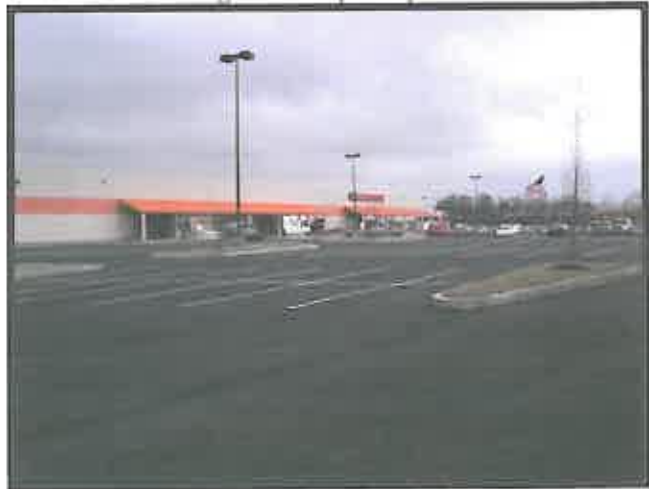
Paving Home Depot Expansion
