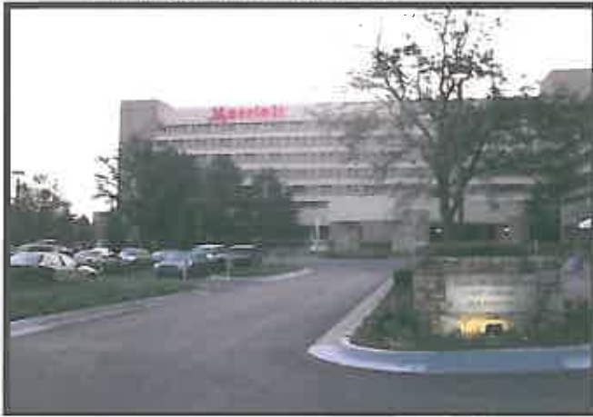
Paving Marriot parking complex
