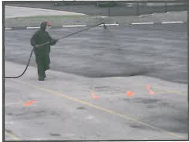
Spraying sealcoat by wand
