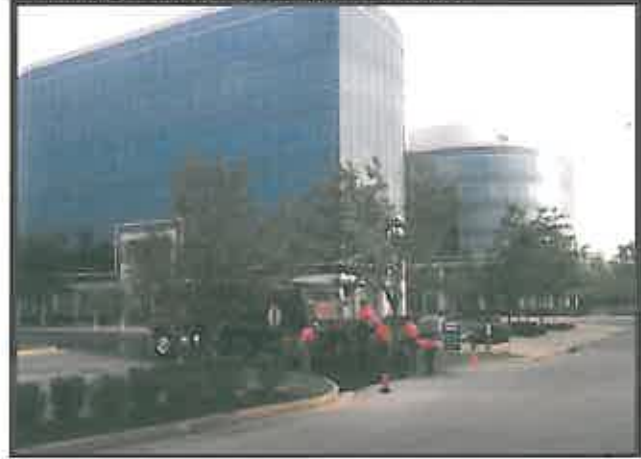
Paving Lexington Green Office Complex
