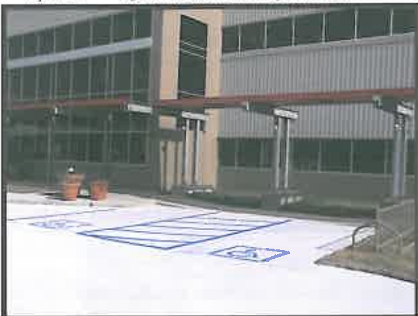
Special UV reflective sealer at Toyota Plant
