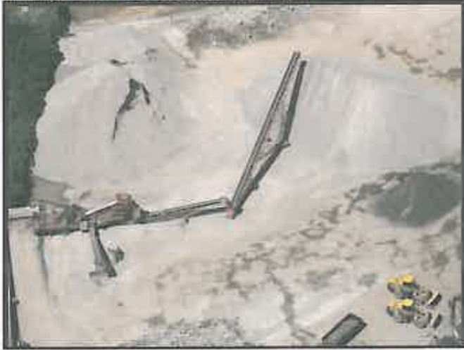
Recycling Yard at C & R Asphalt Complex
