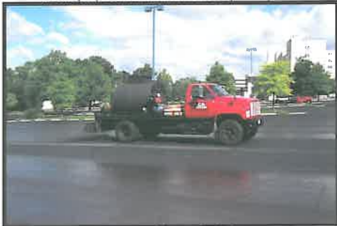
Truck spray bar installation-St. Joseph Hospital
