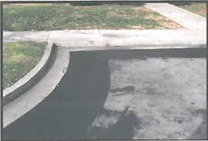
Hand brushing areas adjacent to concrete/brick
