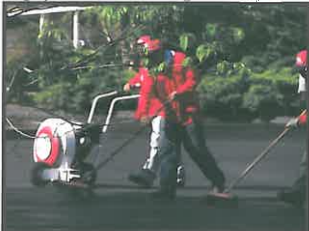
High speed blowers and brushing to clean surface
