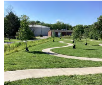
East Hickman Pump Station site.
