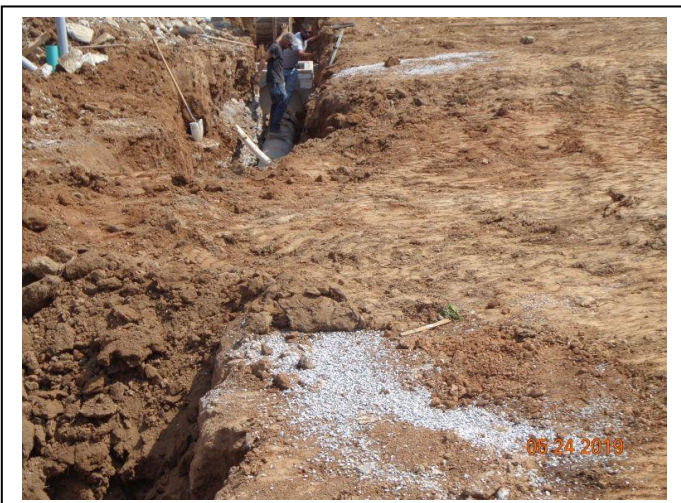
Photo #005 – Str pipe in progress (typical)
