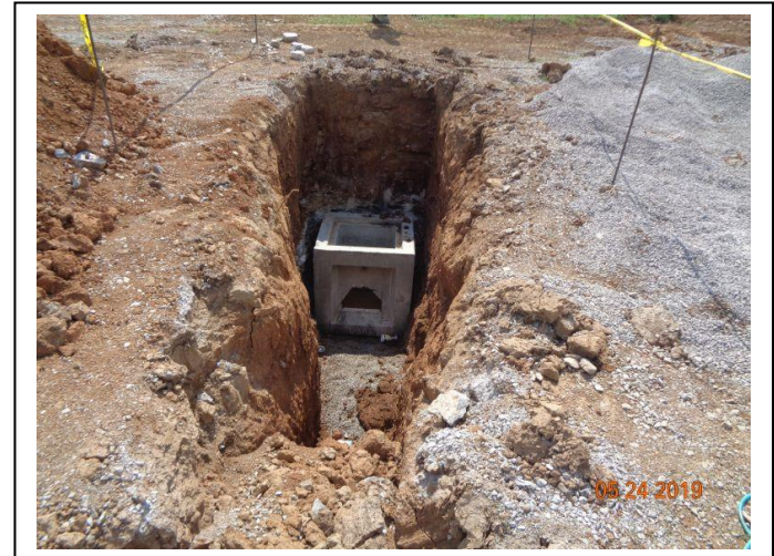
Photo #004 – Catch Basin and work in progress
