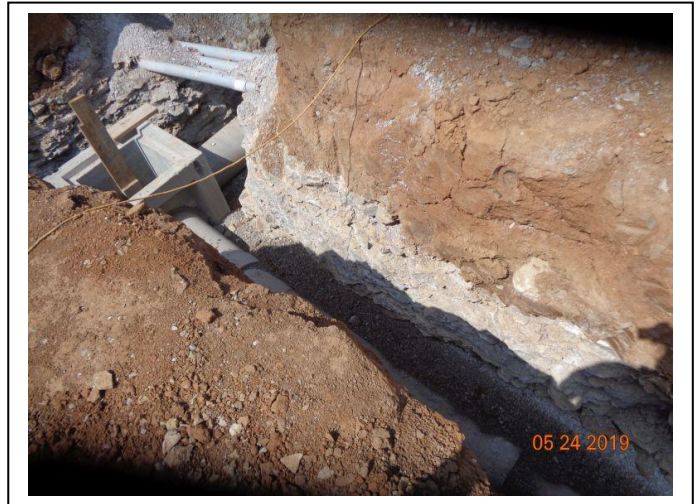
Photo #002 – CB2 to CB4 rock excavation
