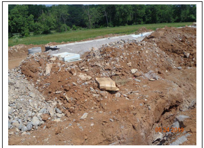
Photo #008 – Rock spoils encountered during Utility excavation (typical)
