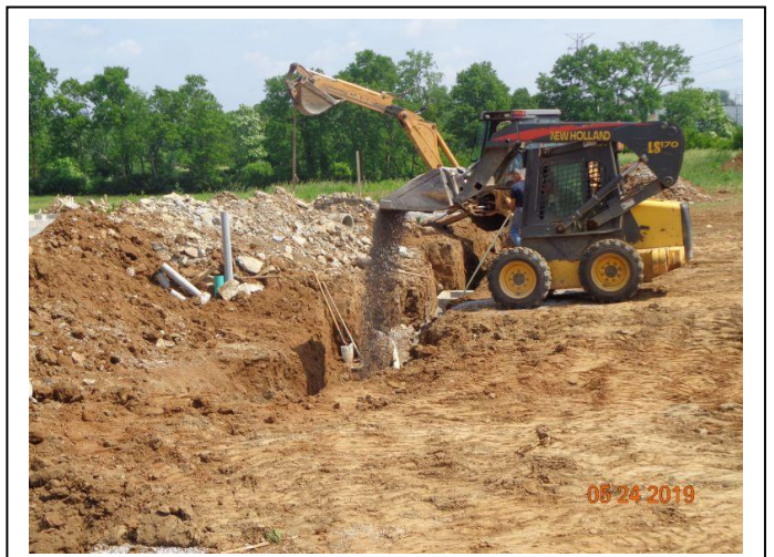
Photo #006 – Backfilling & haunching of Str pipe in progress (typical)
