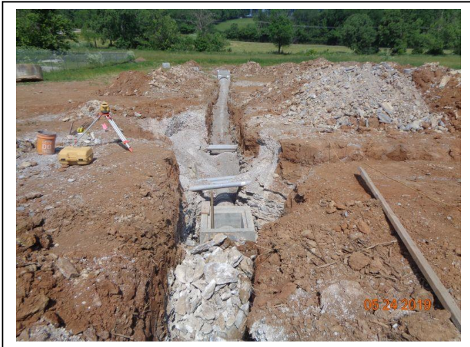
Photo #001 – CB1 to CB2 rock excavation
